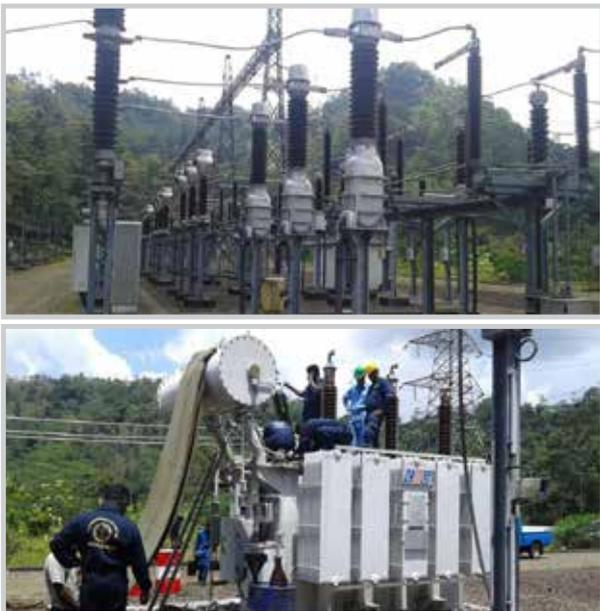
**Servicing of tap changer of 10MVA Transformer at switchyard of KGPS**
