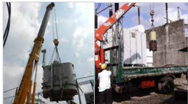
Replacement of defective single phase 250/3MVA 220-132/33kV Transformers at Biyagama GS
