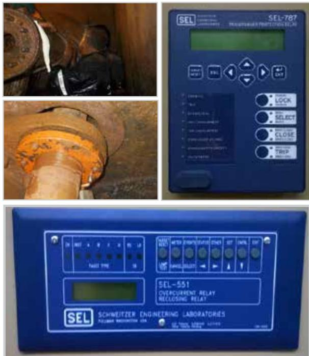
Installation of transformer protection relays (SEL 787 and SEL 551) was carried out by replacing existing electro mechanical relays.
