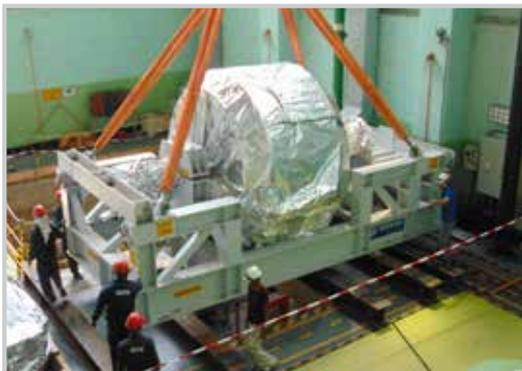
Rehabilitation of the 1st unit at Samanala Power Station commenced on Nov. 2016 and is expected to continue until April 2017. Existing components of unit 1 were removed to make room for the new turbine, runner and Main Inlet Valve of which are being installed.
