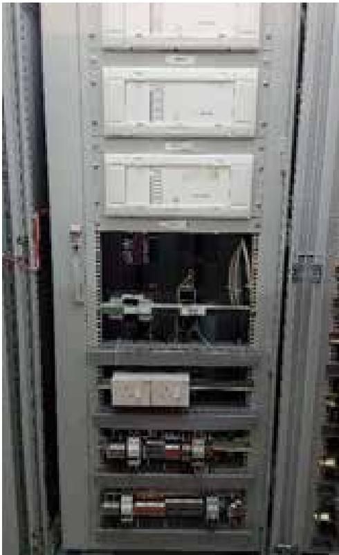
GE 264 RTU Installed at Rantambe Power Station
