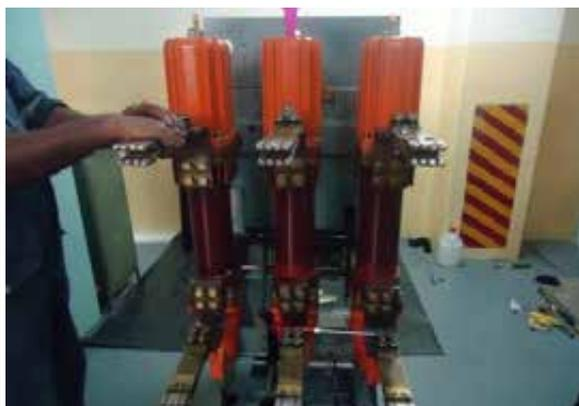
Canyon 12.5KV spare generator OCB overhaul works
