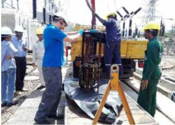
Disassembling a Diverter Switch at Rantembe switchyard
