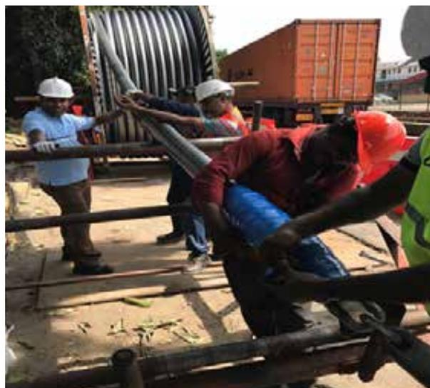
220kV Cable Pulling Work at Port Premises
