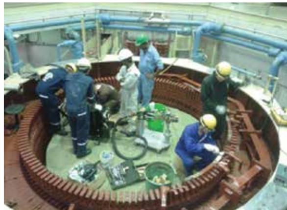
Soldering the replaced Stator Winding Bars in U-1 Generator
