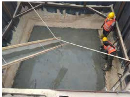
Construction of Tower Foundation Works are in Progress at the site of Mannar - Nadukuda 220 kV Transmission Line
