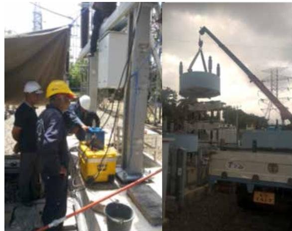
Circuit Breaker Testing at Ampara GS
