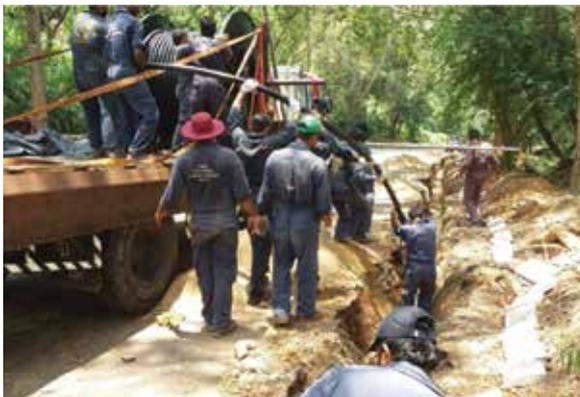
Replacement of Intake 11kV Power Supply Underground Cable at Victoria Power Station
