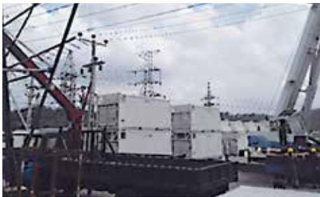
Installation of Containerized 1MW diesel Generator
