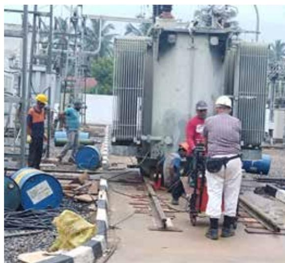
10MVA transformer at Old Anuradhapura GS was replaced with a 30MVA transformer transported from Old Galle GS after complete overhaul and assessment based on electro-chemical test results to improve the capacity of Old Anuradhapura GS.
