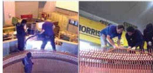
Stator Replacement of Unit 03 Machine at Victoria Power Station
