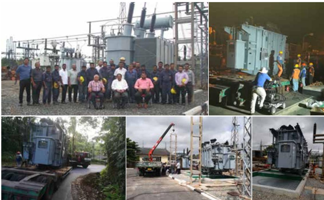
Figure 4: Installation of a new 31.5MVA Transformer at Pannipitiya GS which was shifted from Deniyaya GS.
