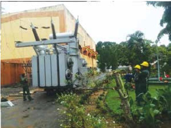
Replacement of Two Generator Transformers at Ukuwela Power Station
