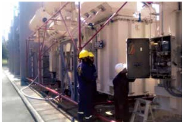
Rehabilitation of Interbus Transformers' Control Panels at Rantembe Switchyard
