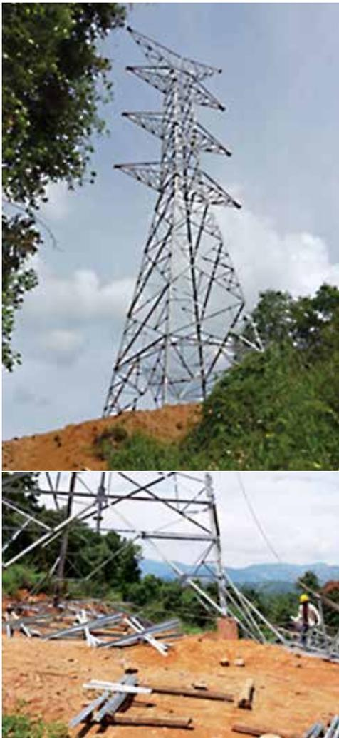
Reconstruction of Badulla - Madagama 132kV Transmission line - construction works
