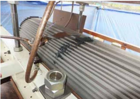
Repair the Core Earthing
