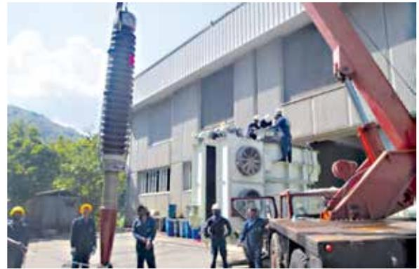
Replacement of Unit 03, 220kV Transformer Bushing at Victoria Power Station
