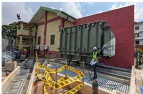
**Figure P 10: Placing 132kV/33kV 31.5 MVA Transformer at Dehiwala Grid Substation.**
