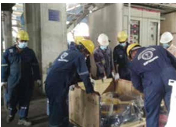
Figure A 8: Replacement work Traction Motor of Lift at Boiler no. 02 - LVPP
