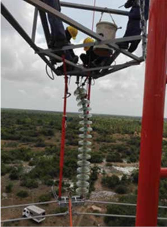
**Figure T 17 : Insulator Replacing in Progress under Hot Condition**
