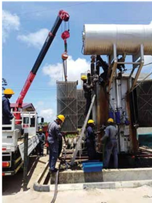
Figure T 16: Transformer Gasket Replacement work at Madampe GS
