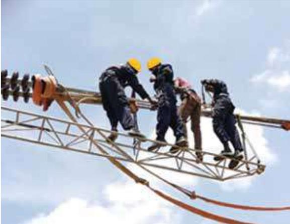
Figure P 15: Padukka- Pannipitiya transmission line stringing works
