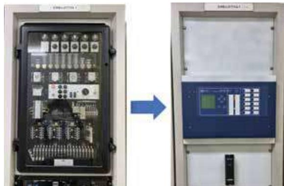
**Figure T 18 : Old Relay and New Relay**
