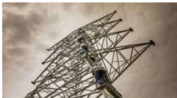
Figure P 5: Erection of 132kV transmission line
