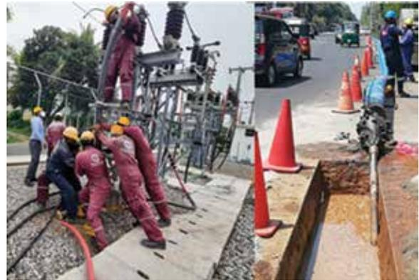
**Figure D 8: Cable laying in progress**
